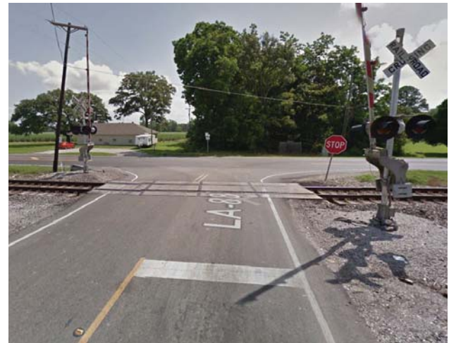
Figure 1 Railroad crossing in close proximity to a roadway intersection
