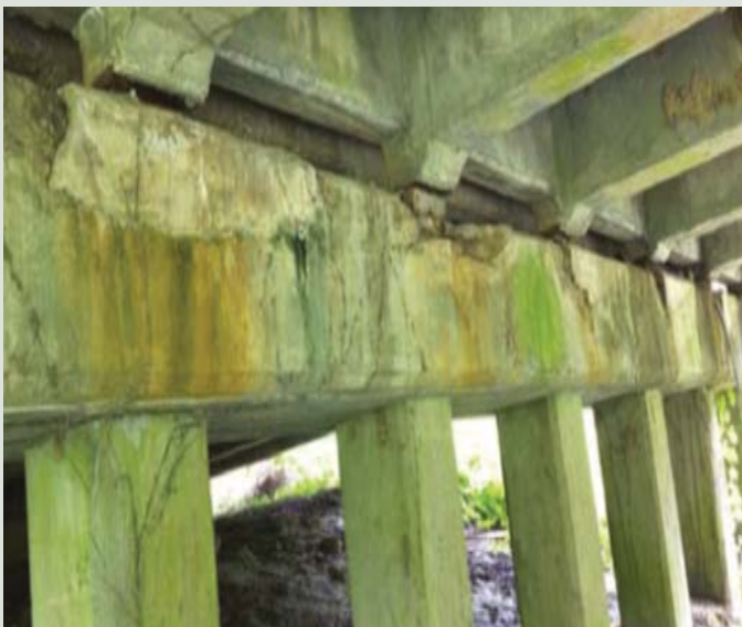
Pier-cap pre-repair: delamination under the bearing plate
