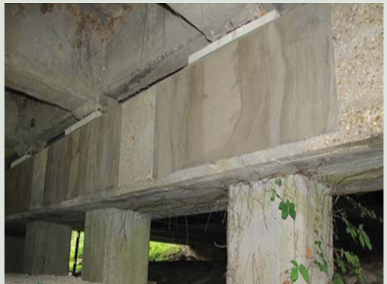
View of the bent after the repair
