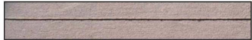
a) No raveling—sawed later in the window
