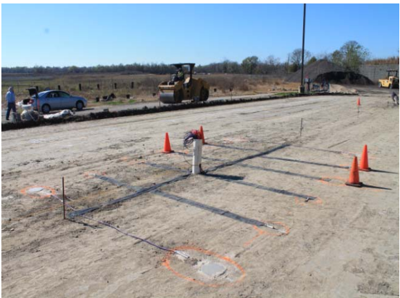
(c) Protecting the wires
