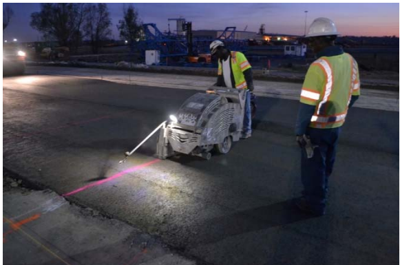
(e) Saw-Cutting Joints
