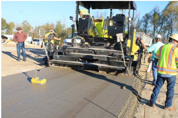
(c) Placement of RCC
