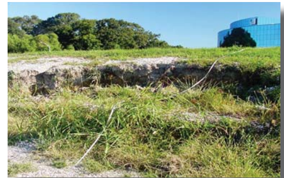
Figure 1 Example of surface sliding failure
