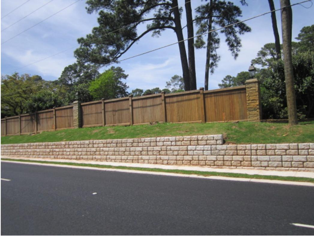
Figure 8. Photo. Completed gravity retaining wall system.
