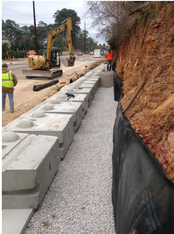
Figure 6. Photo. Unreinforced concrete leveling pad (not shown) with first course of block installed with the stone backfill material shown.
