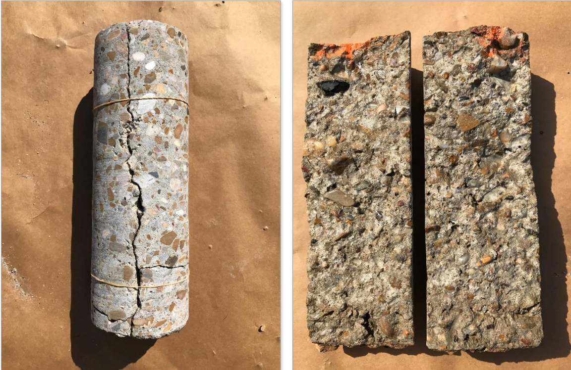
Figure 7: Cores from the Longitudinal Joint
