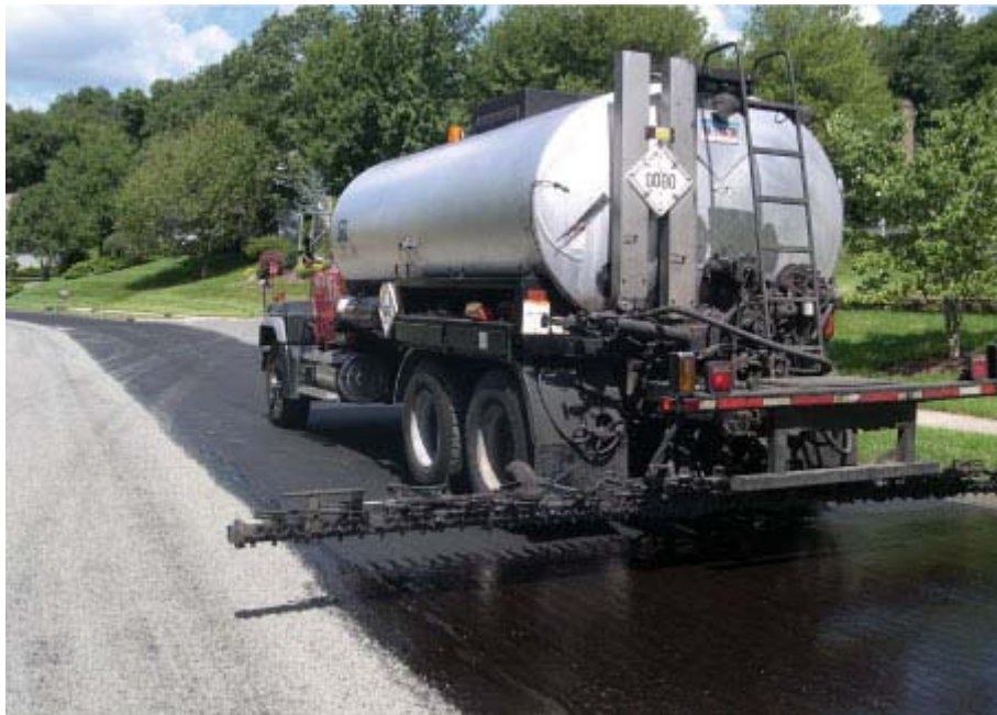
Figure 1 Typical application of tack coat
