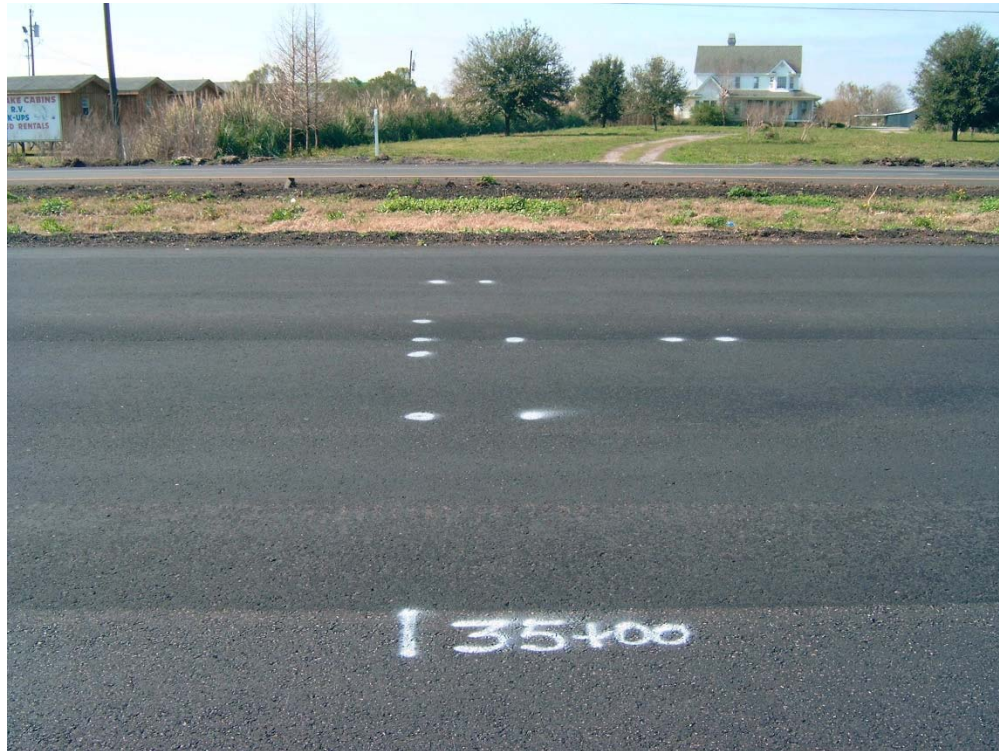
Figure 4 Coring for STA 35+00
