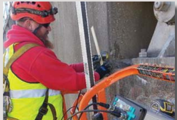
Figure 2 (bottom): FDH operator performing UT measurements
