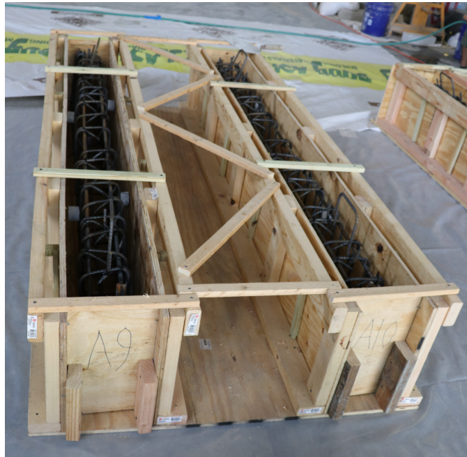
Figure 49. Reinforcement cages placed in the form.
