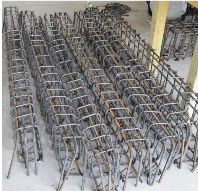
Figure 48. Assembled reinforcement cages.
