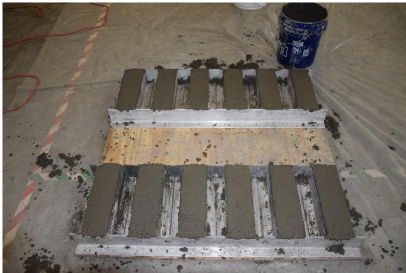
Figure 39. Forms filled with fresh concrete.
