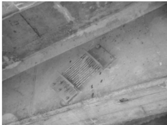
Figure 9. SMA rods installed in a bridge girder in Michigan to control of shear cracks [9].
