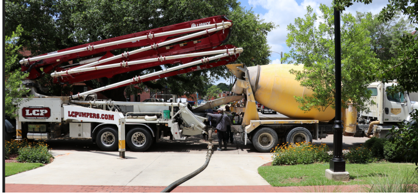
Figure 50. Concrete pumping arrangement.
