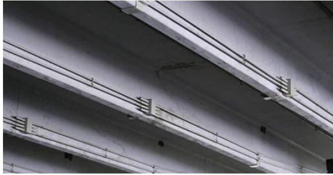
Figure 1. External post-tensioning [Structural Group, Inc. 2016].
