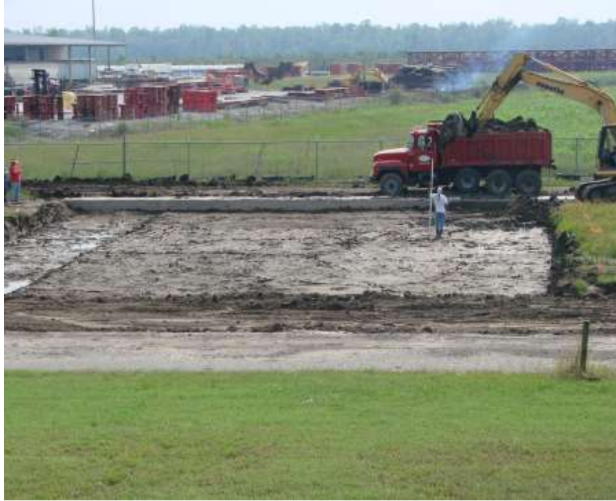
(a) Site preparation
