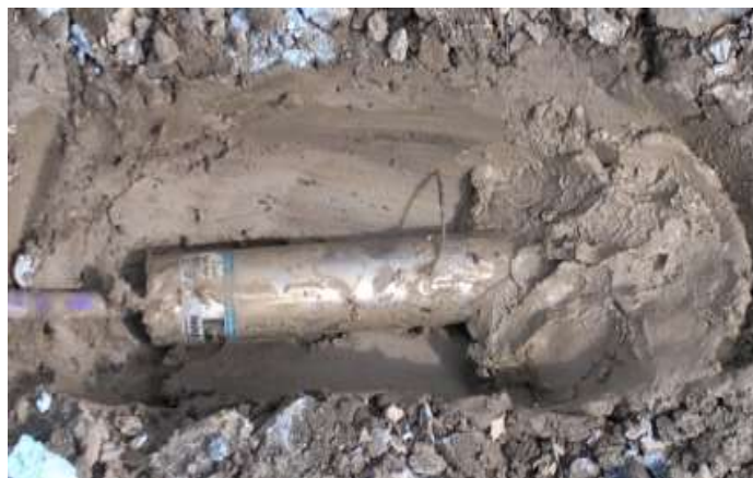
Figure 11 Placement of piezometers
