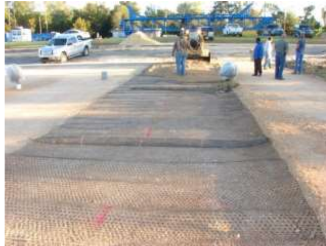
Figure 14 Placement of geogrids with strain gauges
