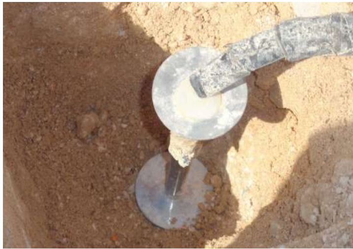
Figure 15 Placement of potentiometers
