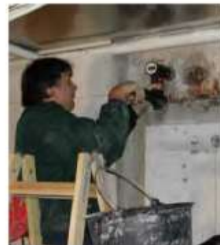
CAPO-TEST being performed in parking garage to evaluate in-place strength of suspect concrete
