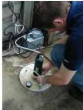
Routing recess for the expandable ring in preparation for CAPO-TEST to evaluate surface strength of an industrial floor slab
