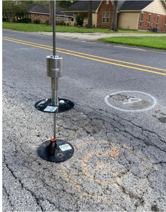
Figure 28. Photo of Zone 10 DCP and core location
