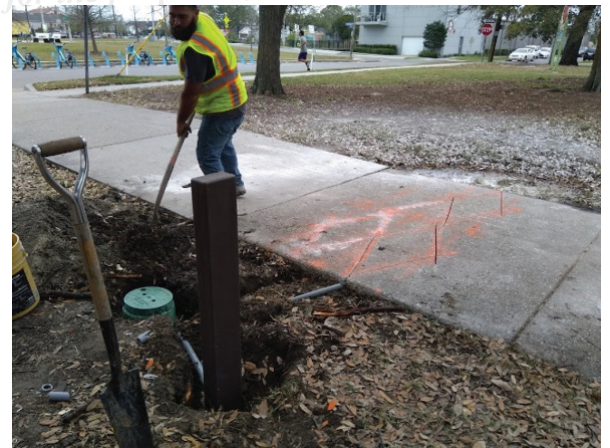
Figure 1. Installation of EcoMulti pedestrian and bicycle counter on Norman C Francis Parkway Trail, New Orleans, March 2020
