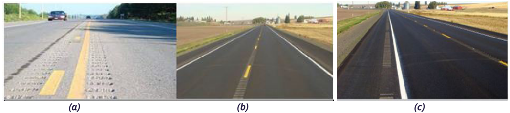
Figure 1. (a & b) Centerline rumble strips (Source: McCully and Briese, 2008 and FHWA, 2018) (c) Shoulder rumble strips (Source: FHWA, 2018)
