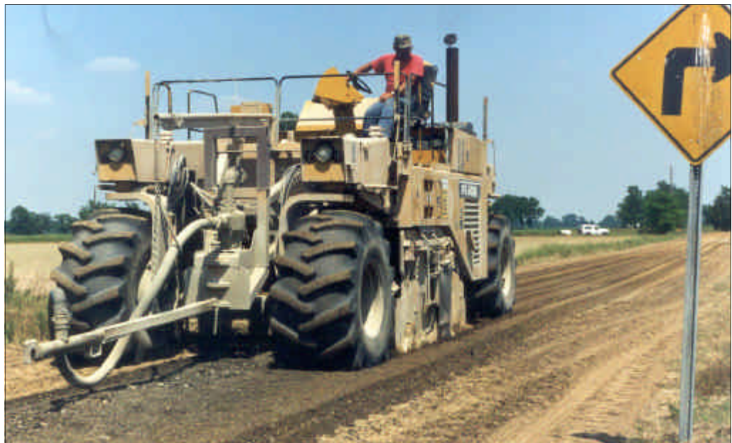
Soil cement project on La. 870 in Franklin Parish.
