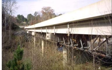
Photo 23: South elevation, exterior Girder E. Note 8-in. sewer pipe below Girders D & E.
