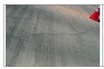
Photo 10: Close up view of the cracks at deck joints.
