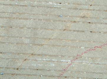
Photo 9: Close up view of typical longitudinal crack.
