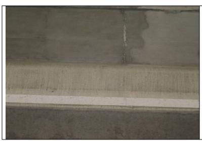
Photo 10: Cracks with efflorescence along the overhang on the westbound bridge.
