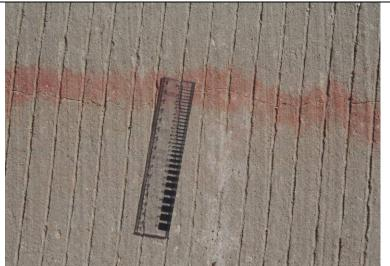
Photo 7: View showing typical crack in the bridge deck. Crack width is less than 1/32 in. and is categorized as hairline.
