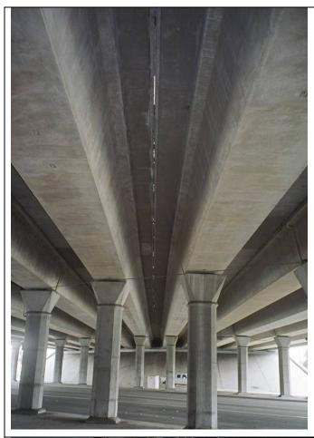
Photo 4: View showing bridge substructure consisting of U-beam girders and columns. Separation between northbound and southbound bridges is shown at the center.
