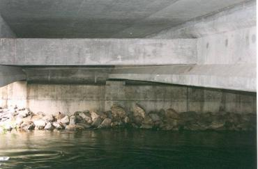
Photo 5: Close up view of bridge deck underside inspection using a boat.
