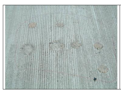
Photo 10: Failed patching work on bridge deck.
