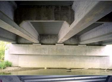
Photo 17: View of the girders A through E, Span A, Pier 1 (fascia girder A is on the left).
