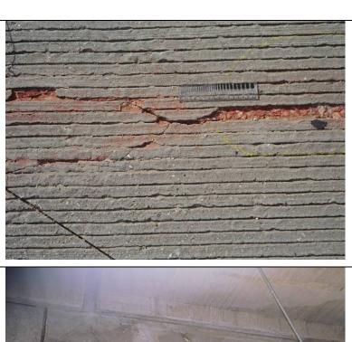
Photo 8: View showing spalling associated with cracks in the deck at span ends.
