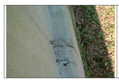
Photo 13: Close up view of the settlement related cracking at the eastern end of bridge Span 5.
