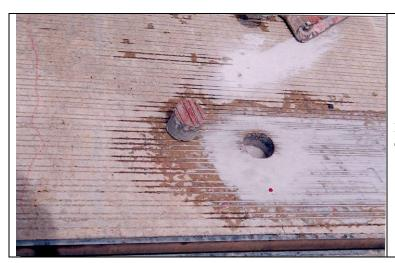
Photo 13: View of the drilled cores on bridge deck.
