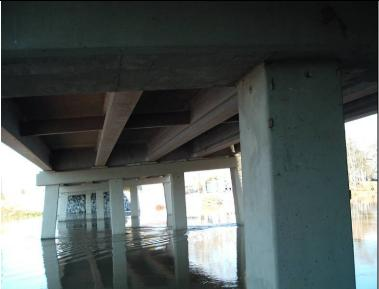
Photo 5: View of the underside of bridge, the pier in foreground supports Span 4.
