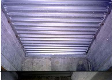
Photo 16: View of the underside of the deck showing the stay-in-place forms.
