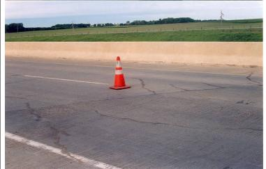
Photo 3: Cracks on the north side approach slab on the I-29 Northbound Bridge.
