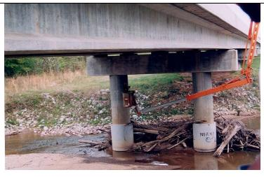
Photo 7: Close up view of bridge deck underside inspection using a snooper.
