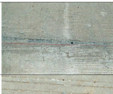
Photo 8: Close up view of typical transverse crack at deck joints.
