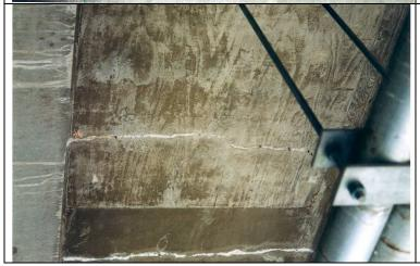
Photo 6: Close up view of the cracking at underside of bridge deck.
