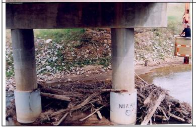
Photo 6: General condition of the piles at Span 2 east facing bridge. Accumulation of debris observed near the pile.
