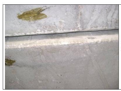
Photo 11: Close-up view showing of the impact crack in the 16<sup>th</sup> girder.
