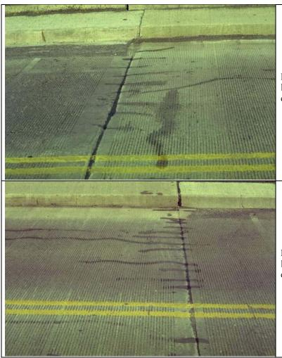
Photo 4: General view of the longitudinal cracks at the south end of the bridge.
