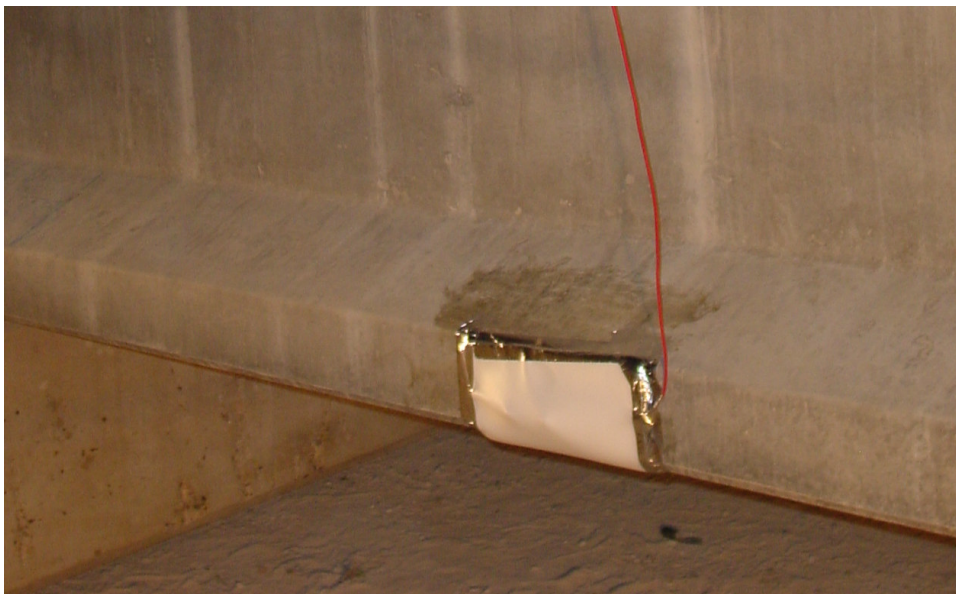
Figure 6 Completed gage cover over gaged area.
