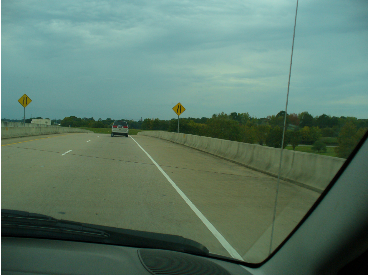
Figure 100 Example of a bridge crossing.
