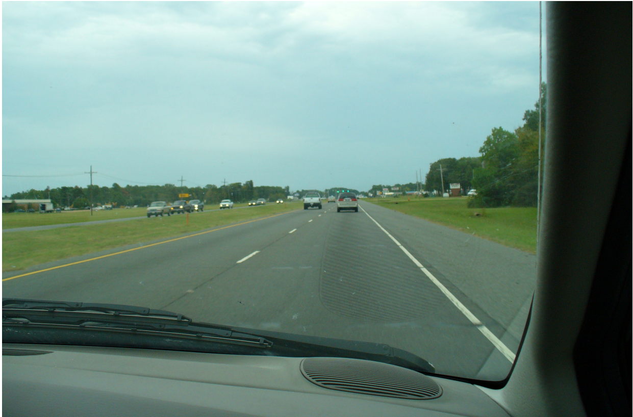
Figure 91 Example of rough road. Note the tar line on the right side of the picture.
