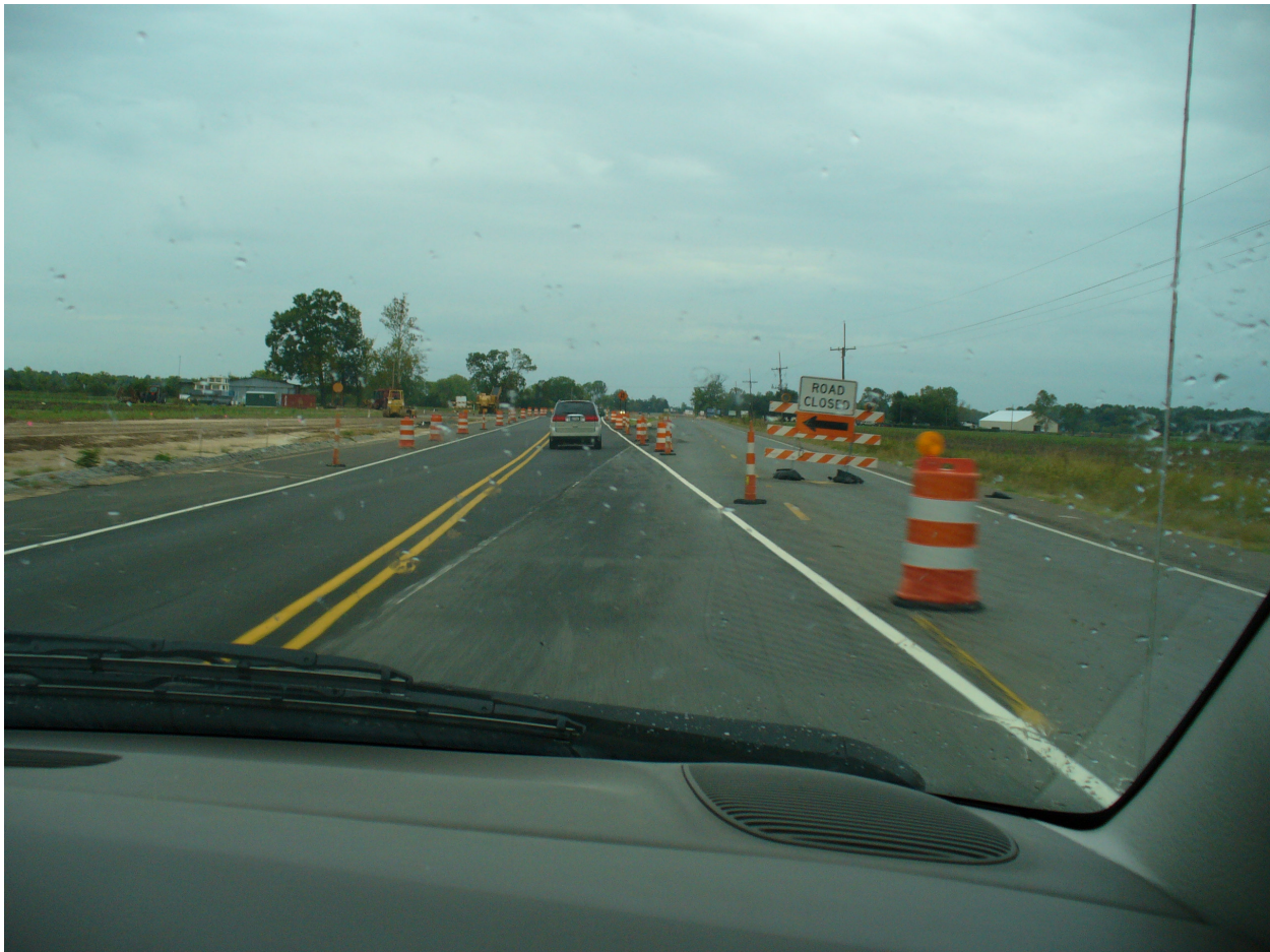
Figure 94 Sample construction zone picture. Median crossings, such as this one, had severe changes in super-elevation.
