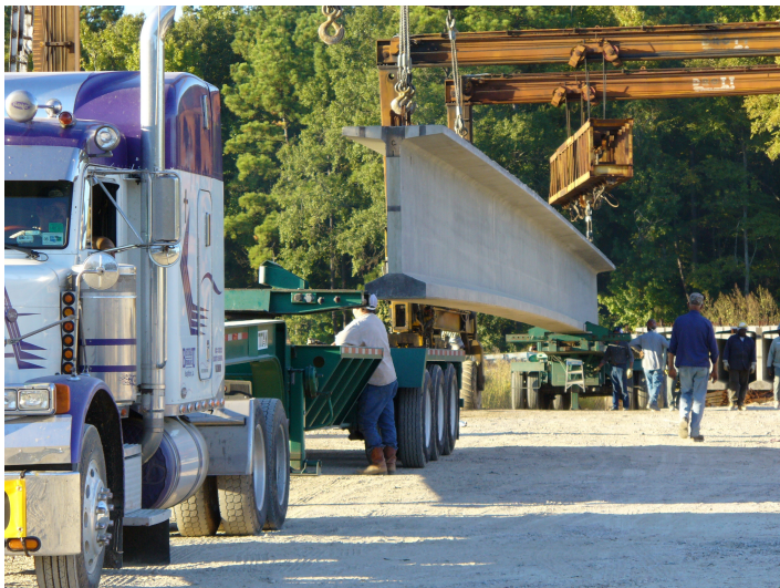
Figure 17 Girder A being loaded onto semi trailer.
