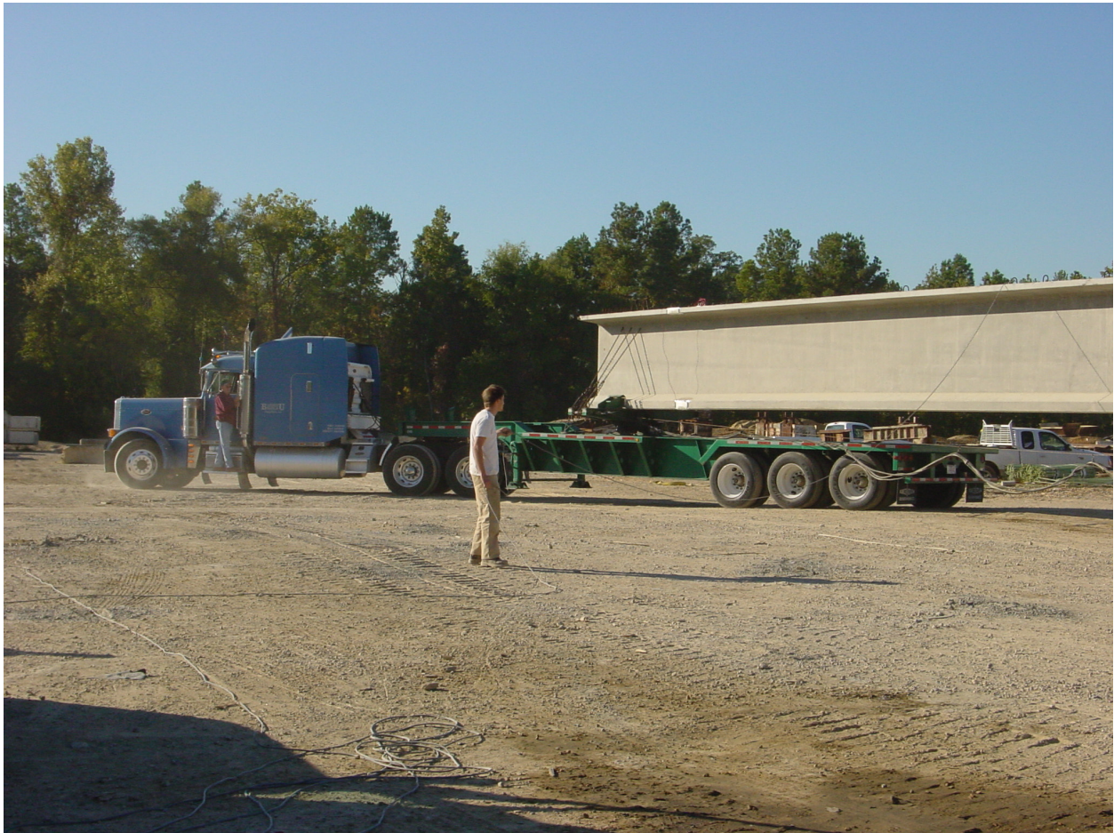
Figure 28 Girder A making left turn to staging area.
