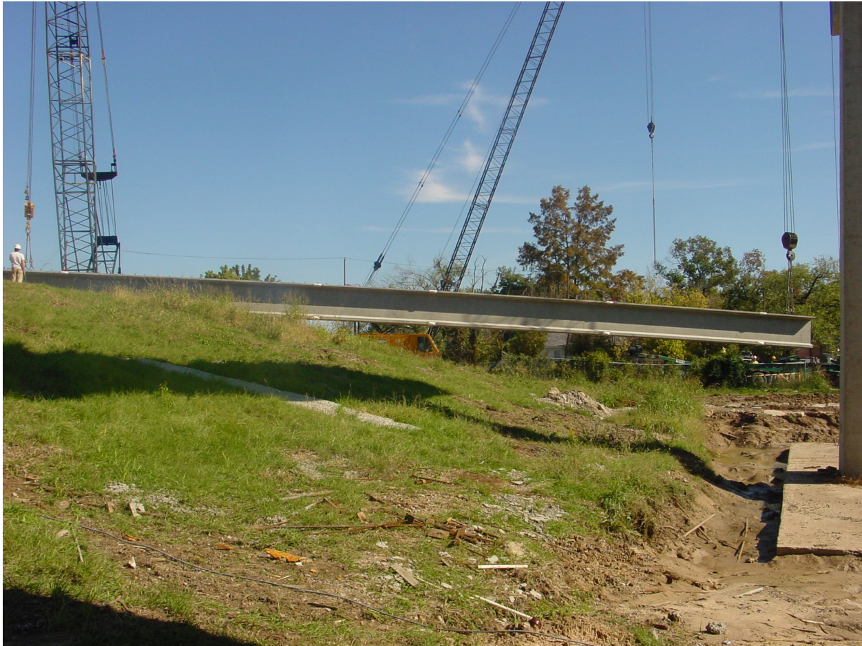
Figure 103 Girder A being hoisted from trailer.
