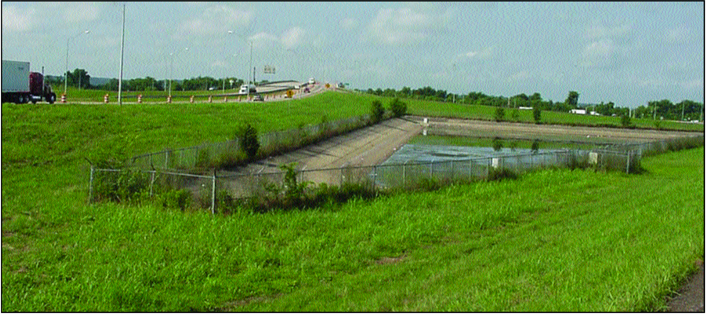
Stormwater treatment pond at highway interchange
