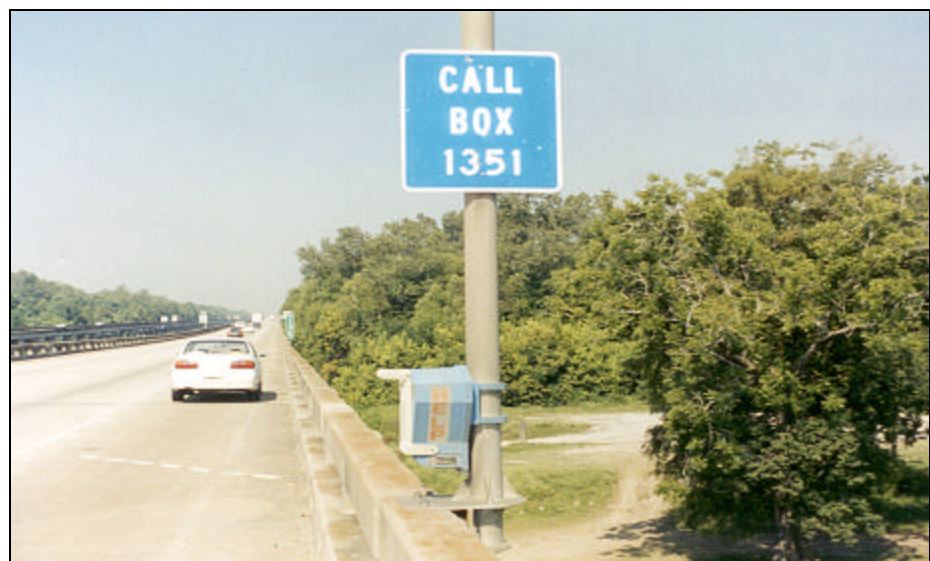
The Louisiana Department of Transportation and Development currently uses a simple push-button call box.
