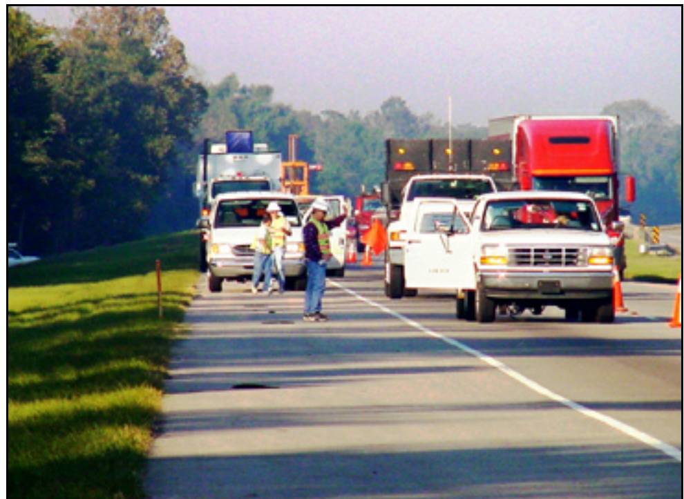
Congestion in the work zone.
