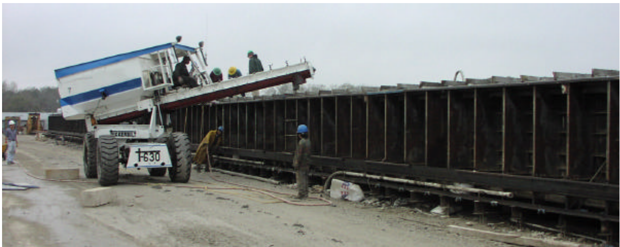
Figure 2 Girder fabrication
