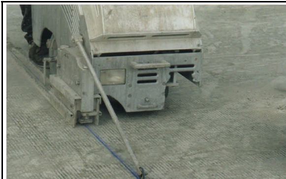
Creating a transverse joint using the saw cut method.
