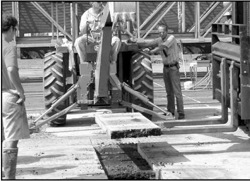
NOT A GRAVE: Bill King, assisted by Glen Gore removes a slab of pavement.
