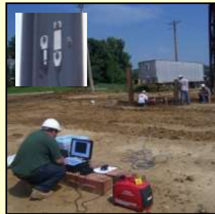
Dynamic Pile Test
