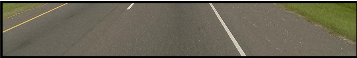
The Louisiana Department of Transportation & Development ©2009 This Asphalt right and left shoulder would be listed as a ASP on the Shoulder Type Table and both left and right on the Side of Road Table
