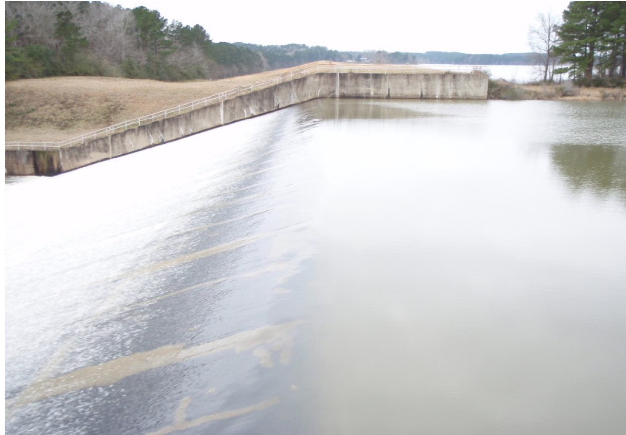
Vernon Lake Dam – Vernon Parish
