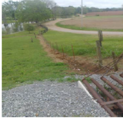
Fig. 2: 0024100m, Fence Crossing Levee
