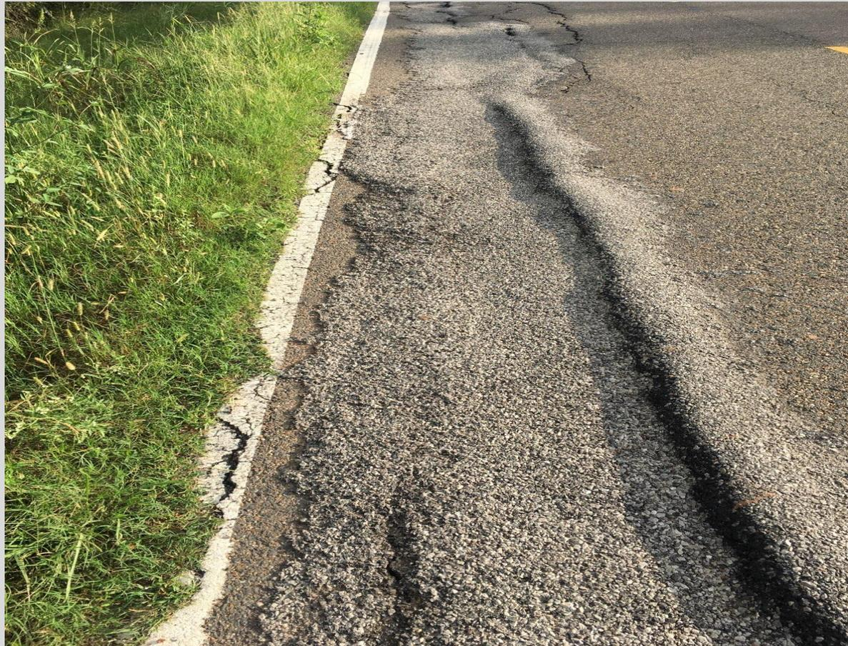
**LEVELING CAN CORRECT FAULTING, BUT . . .
