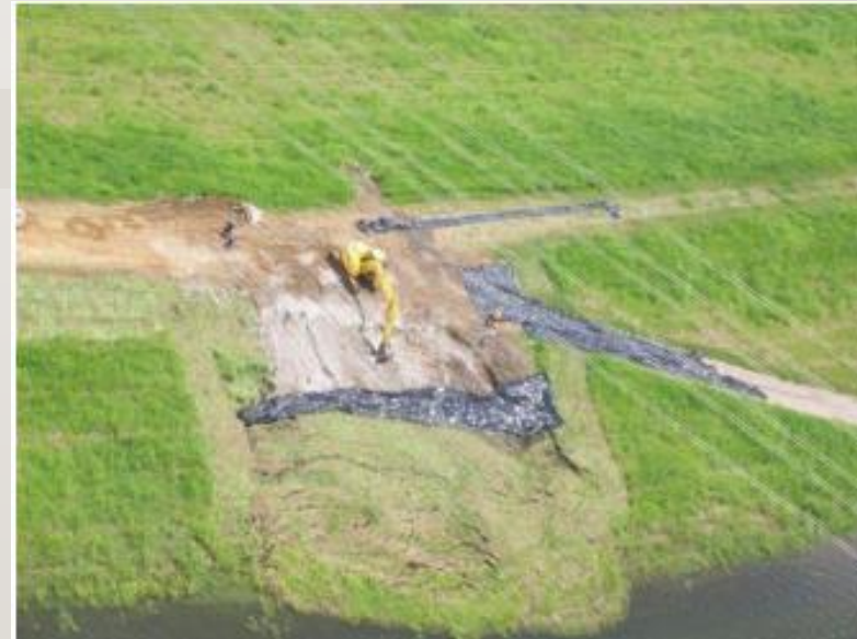
Typical shallow slides in Dallas levees (photograph used with permission from Gamez and Stark (2014))
