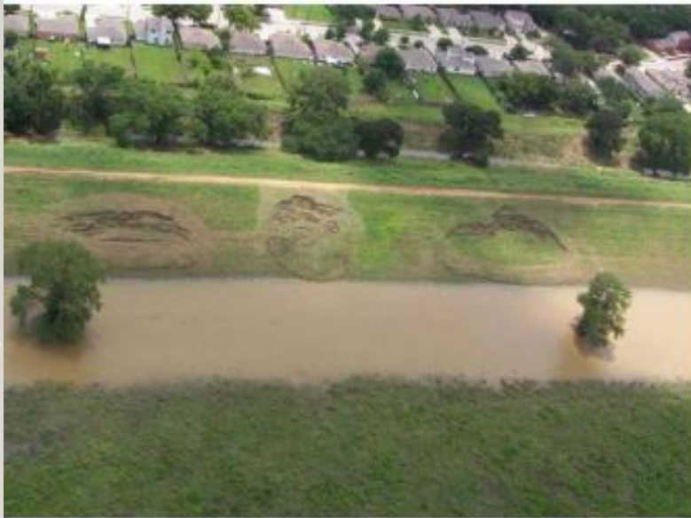
Typical shallow slides in Dallas levees (photograph used with permission from Gamez and Stark (2014))
