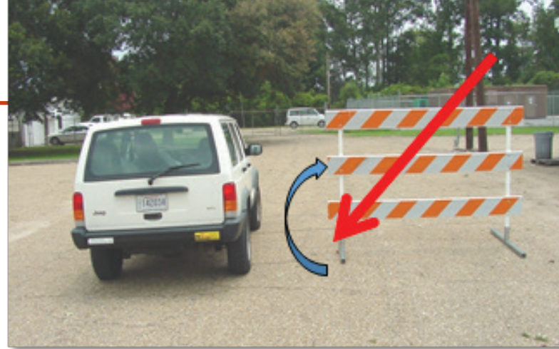
The diagonal stripes on a Type III barricade should slant down and toward the direction on which traffic is to pass.
