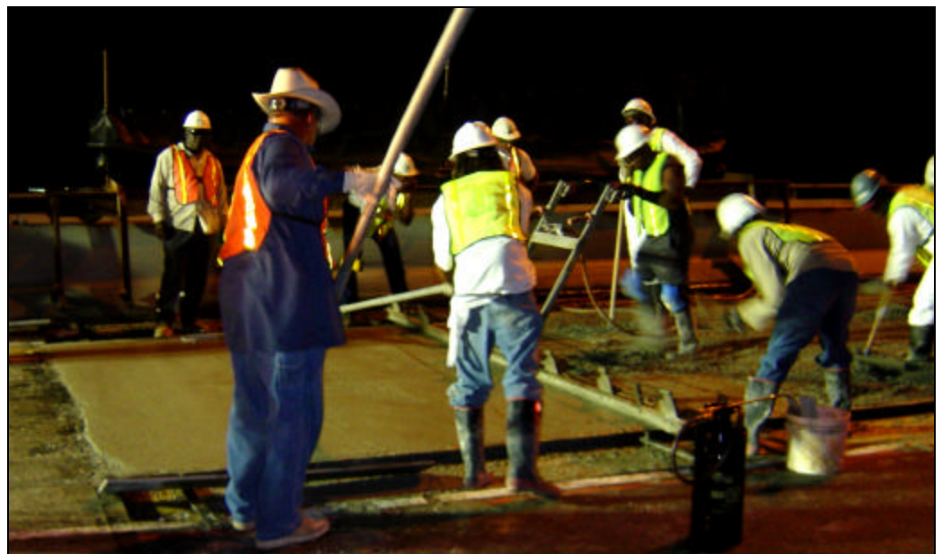
SFRC application on the Luling Bridge deck (9/26/2004)
