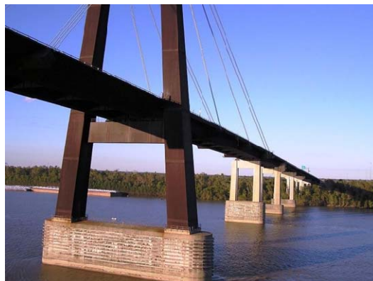
Figure 1 The Luling Bridge (The Hale Boggs Memorial Bridge)
