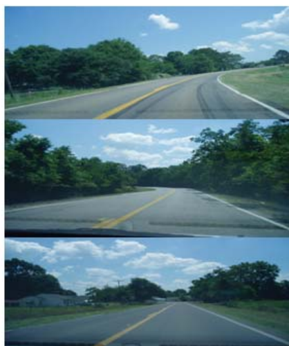
Locations before and after edgelines implementation (pictures taken from different travel direction)
