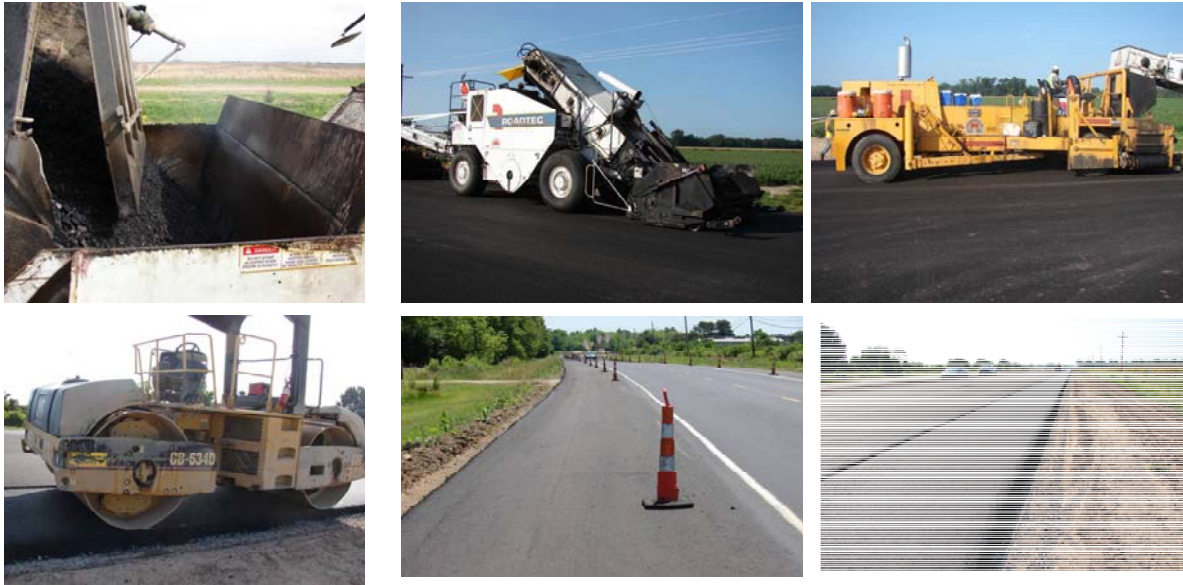
Figure 14 Construction of asphalt treated mixtures layers
