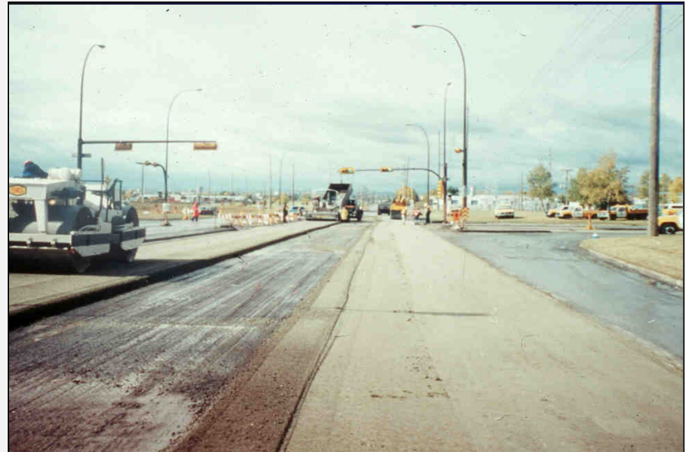
Intersection replacement Calgary, AB
