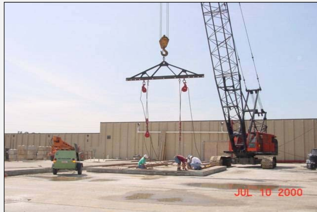
RCC used as working platform for cast-in-place tilt-up walls
