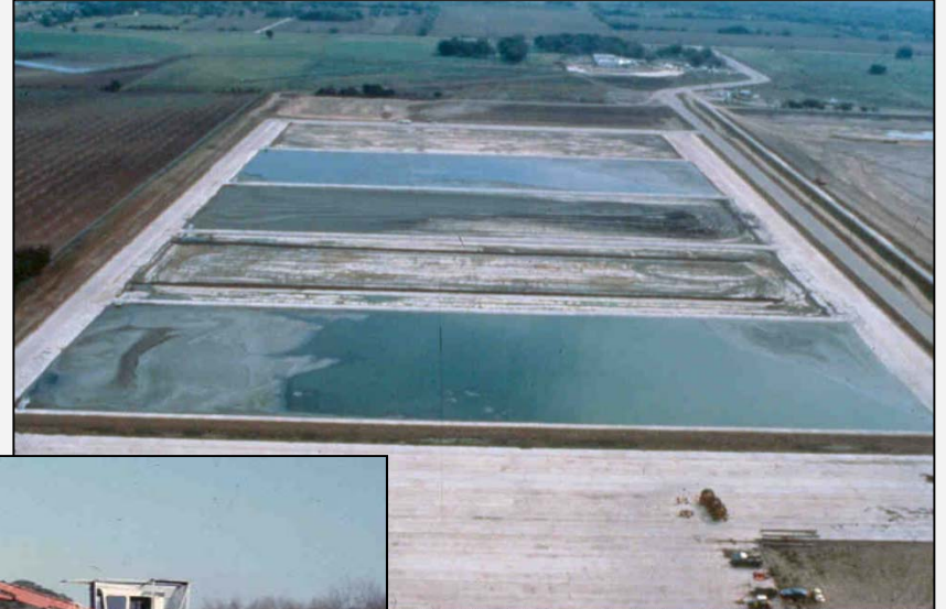
25 acre sludge drying basins in Austin, TX
