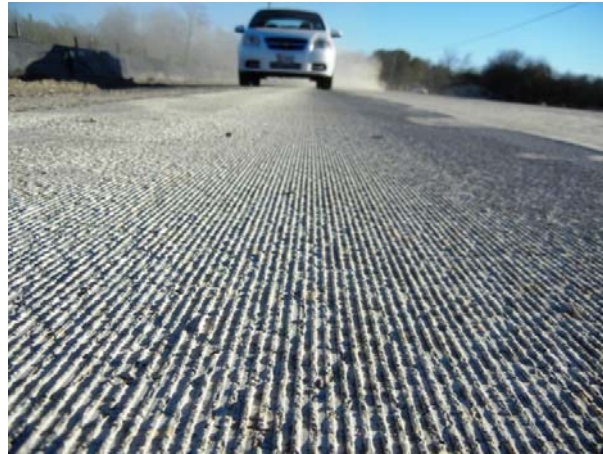
Diamond Ground RCC
