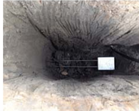
Installation of Moisture gage
