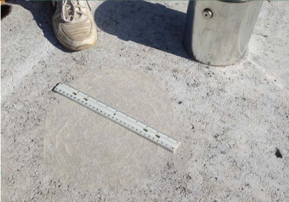
Sand Patch Test for Macro-texture
