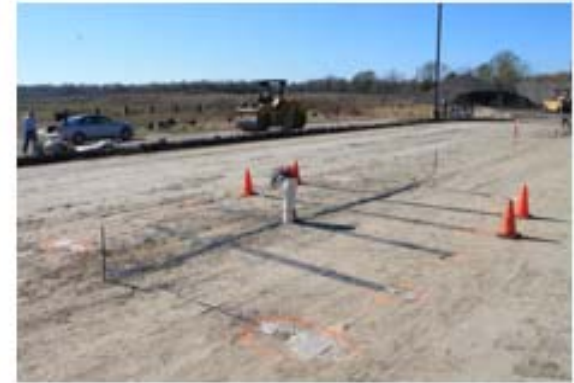
Protecting the Cables
