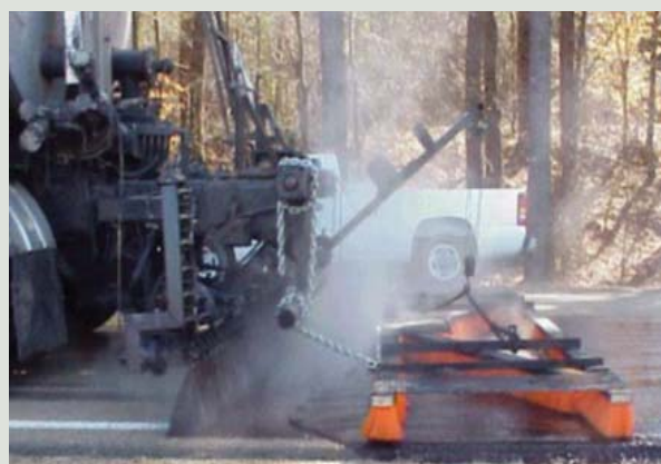
Figure 1 Application of scrub seal (Howard, 2009)
