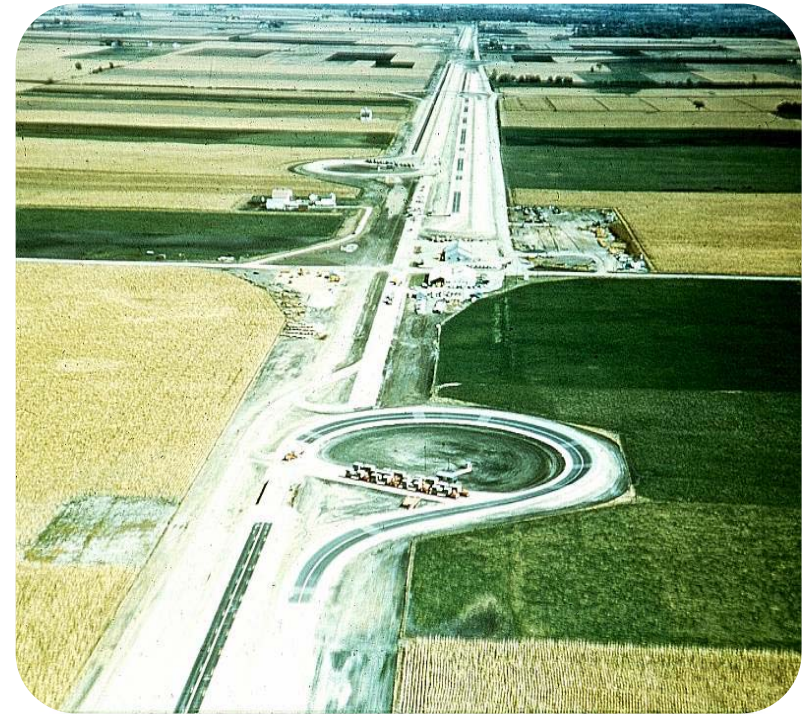
AASHTO Road Test at Ottawa, Illinois (approximately 80 miles southwest of Chicago) between 1956 and 1960
