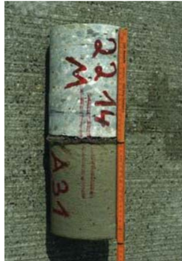
Core from Germany showing non-woven geotextile interlayer between surface concrete and cement-treated base. Fabric bonds to PCC but not CTB or LCB.
