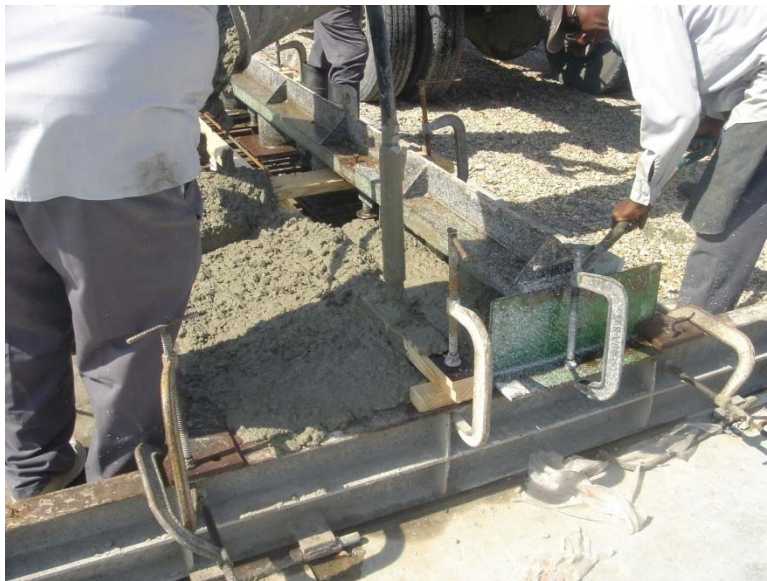
Figure 35 Pouring of concrete in the formed slab frame
