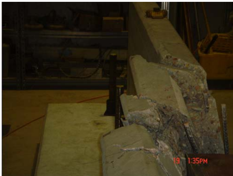
Figure 78 Torsional failure of barrier
