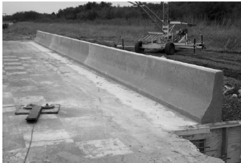
Figure 9 Florida Jersey safety shaped bridge railing
