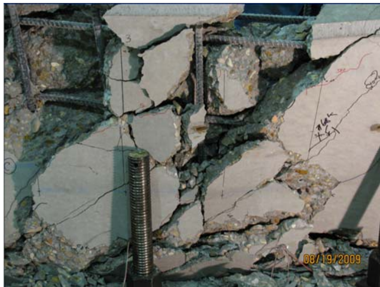
Figure 68 Frontal view of vertical face yield failure
