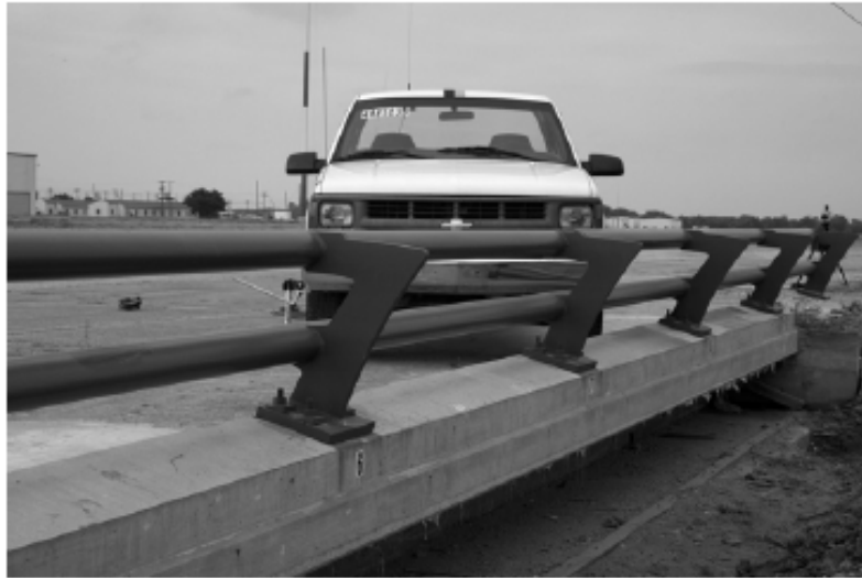
Figure 7 Modified T77 bridge rail before test
