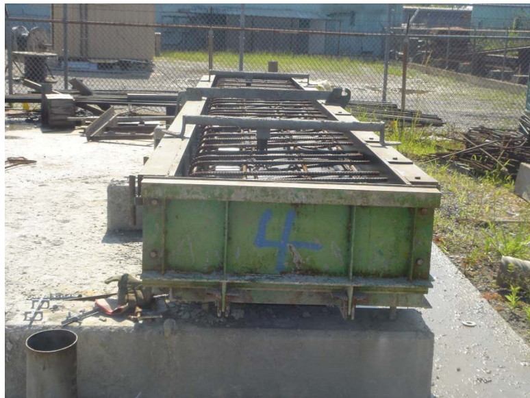
Figure 33 Concrete barrier's form and reinforcement
