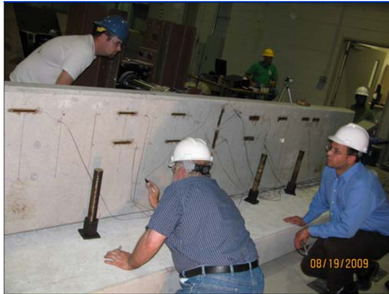
Figure 62 Checking and marking cracks
