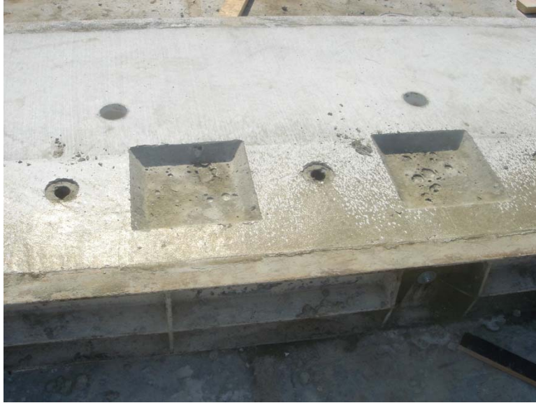
Figure 38 Shear key formed in base of slab
