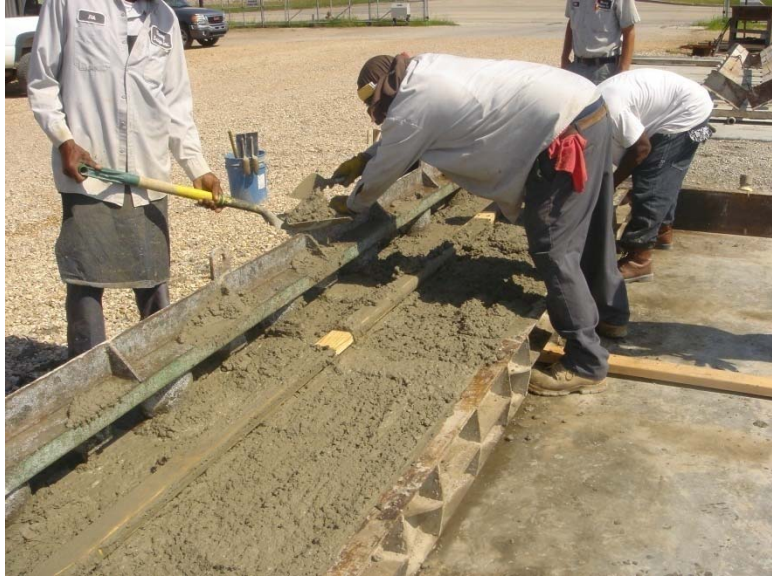
Figure 36 Working of the placed concrete
