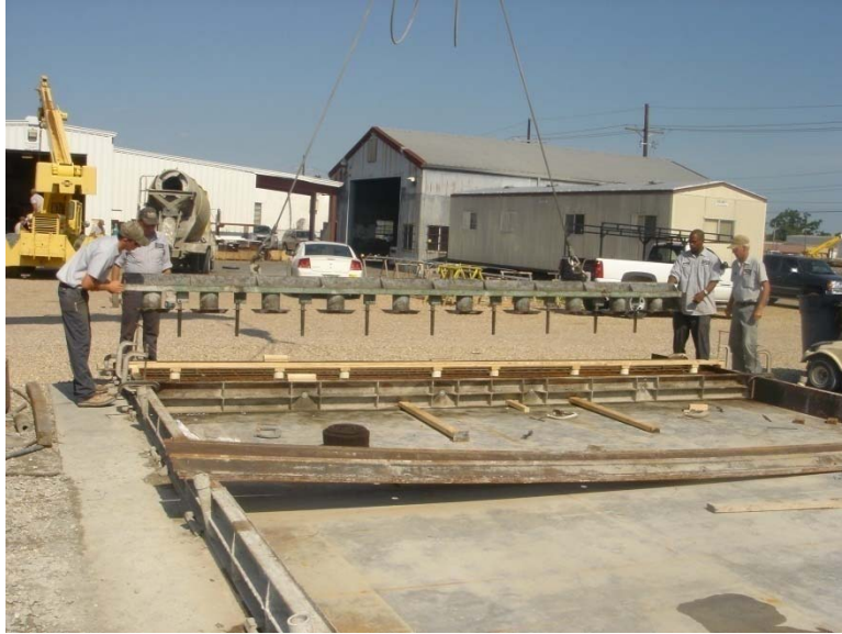
Figure 34 Placement of the special form to create the shear key base
