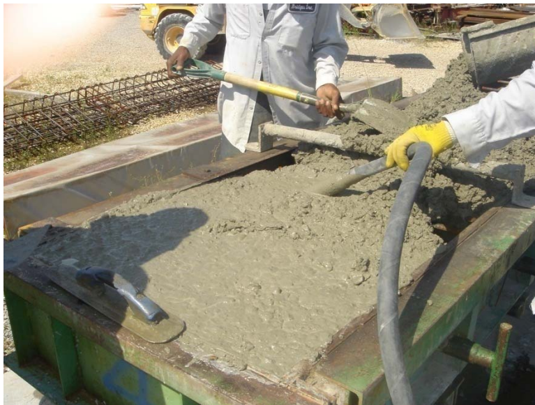
Figure 39 Placing and vibrating the concrete in barrier wall
