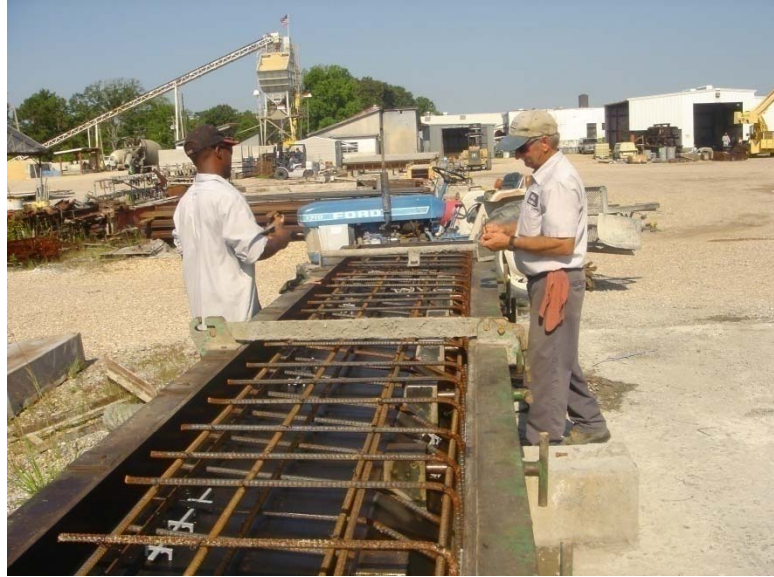
Figure 32 Placement of the reinforcement for concrete barrier
