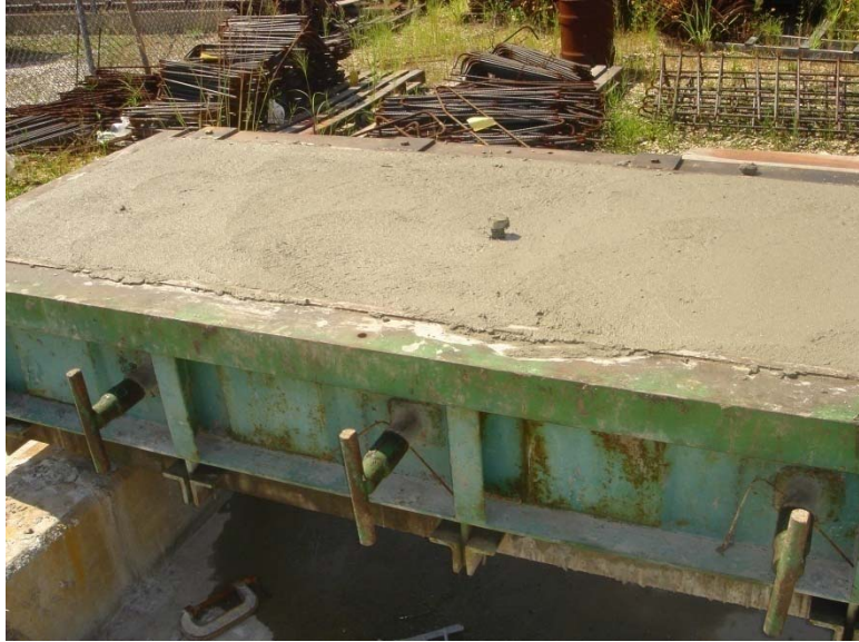
Figure 40 Barrier wall poured
