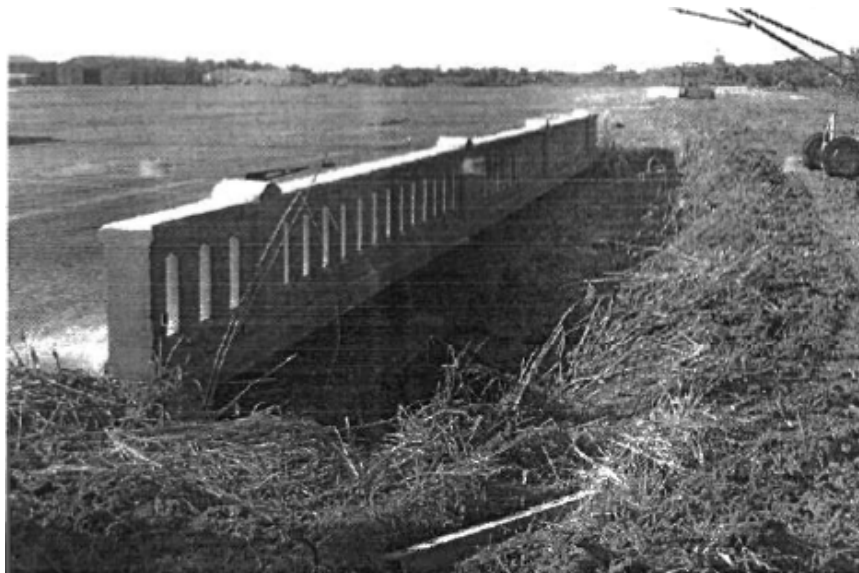
Figure 4 Texas Type T411 bridge rail section
