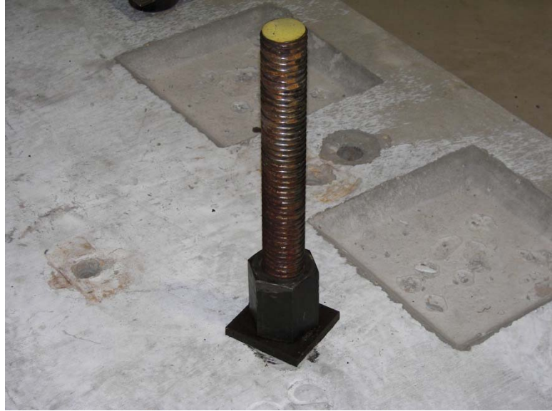
Figure 44 Typical bolt used to anchor slab to strong floor
