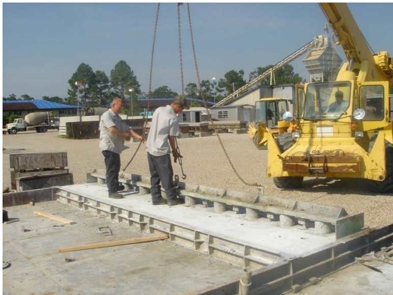
Figure 37 Removing of the block-out form
