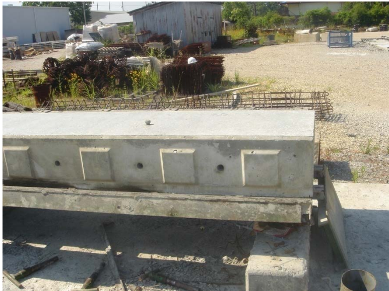
Figure 41 Bottom of concrete barrier
