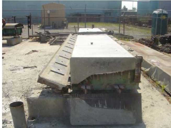
Figure 42 F-Shape concrete barrier after the forms were removed
