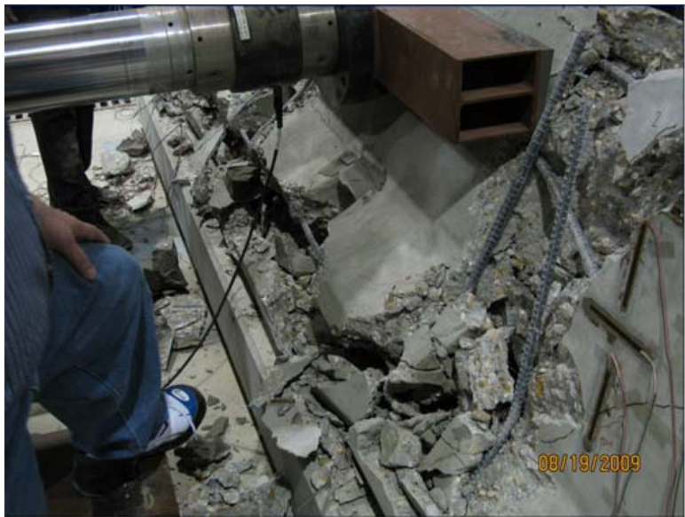
Figure 74 Close-up of cracked region of barrier (sloping face)
