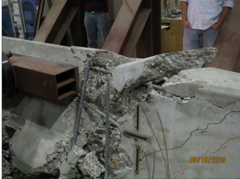
Figure 73 Cracked region of barrier (sloping face)
