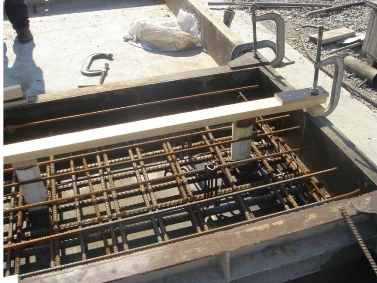
Figure 28 Slab reinforcement is placed in the casting bed
