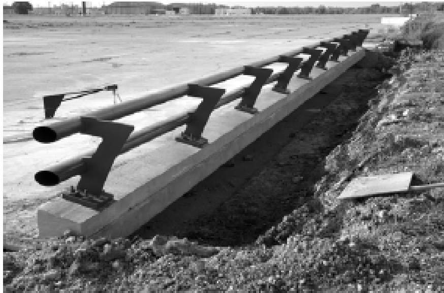
Figure 6 Texas T77 bridge rail
