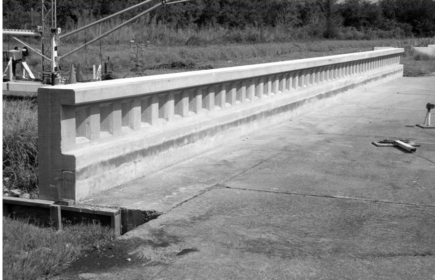
Figure 5 Texas Type F411 bridge rail section
