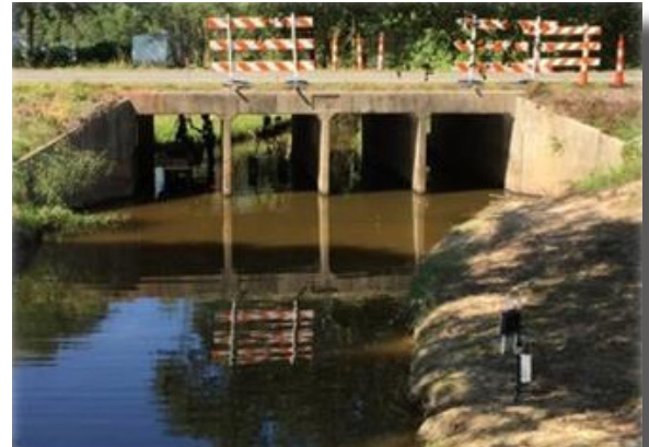
Figure 1 One of the cast-in-place box culverts analyzed in LTRC 16-3ST project
