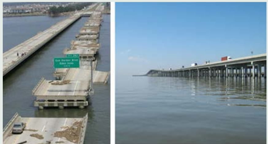
Figure 1 Damaged original twin span (left) and the new twin span (right)
