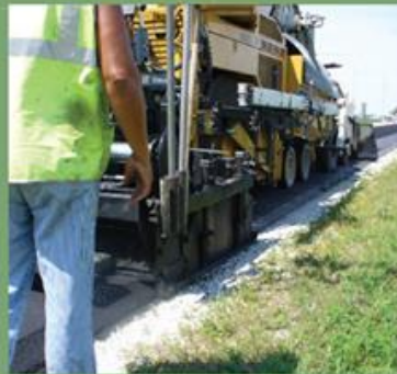
Safety Edge treatment being applied during an asphalt overlay.
