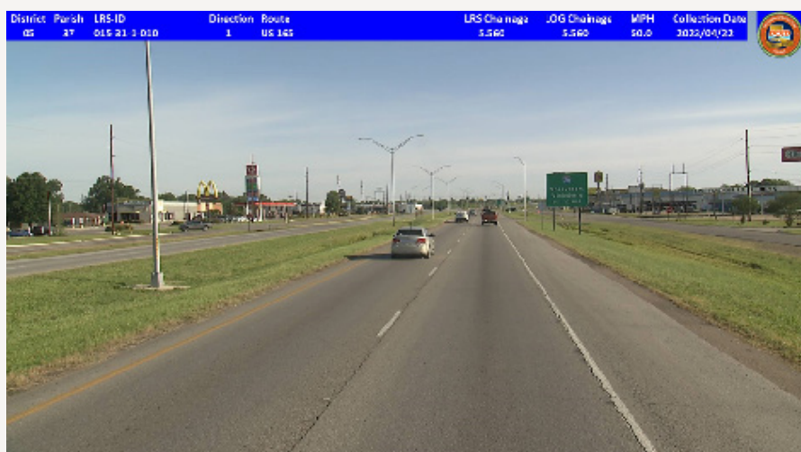
Figure 1. One example of a successfully performing pavement section: overlay of US 165 in Monroe, Louisiana, with an ADT of approximately 40,000
