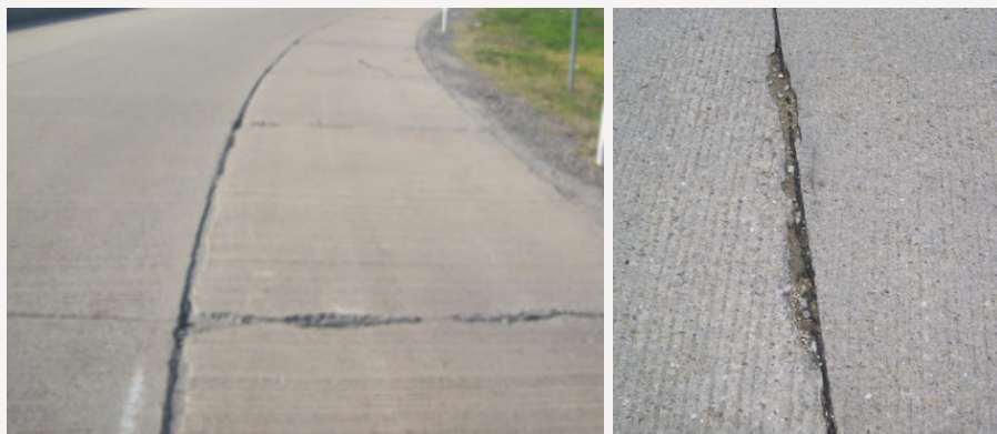
Figure 1. Examples of joint deterioration
