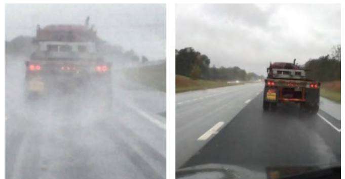
Figure 1. Typical Dense-Graded Mixture (left) vs. OGFC (right)
