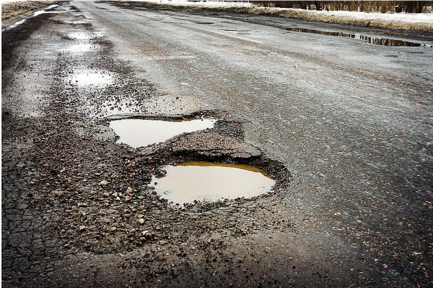
Figure 2. Potholes
