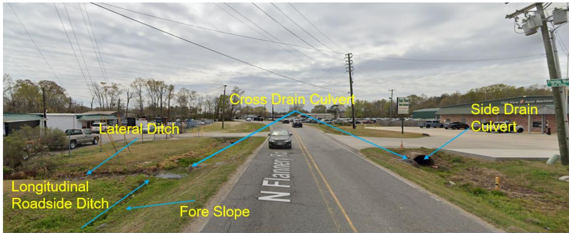
Figure 9. Roadside drainage components
