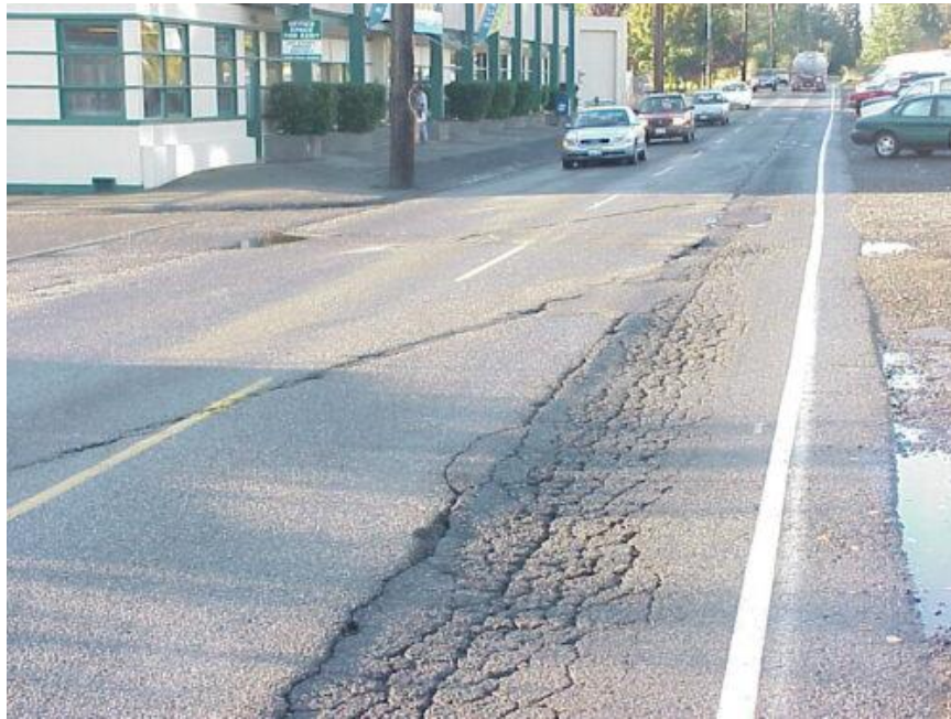
Figure 1. Weakening of base, subbase, or subgrade
