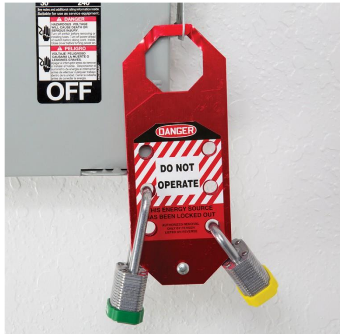
Figure 1.5: Lock Out Power Before Working on Equipment
