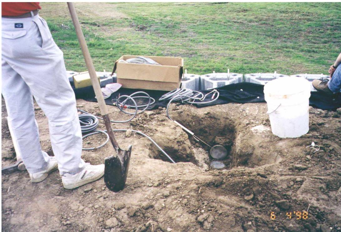
Figure 5 - Installation of earth pressure cells behind the wall facing
